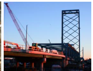
Construction Proceeding on Memorial Bridge (DOT photograph)
