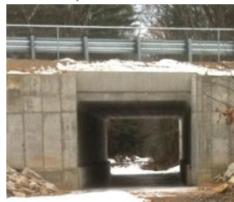
Box Culvert under Route 109 MDOT project. (Photo by Jim Bucar)
